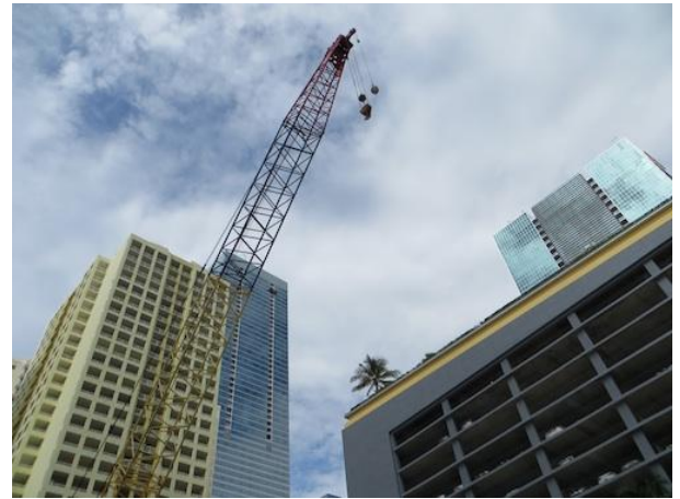
Miami's newest crane rises at the BrickellHouse site
